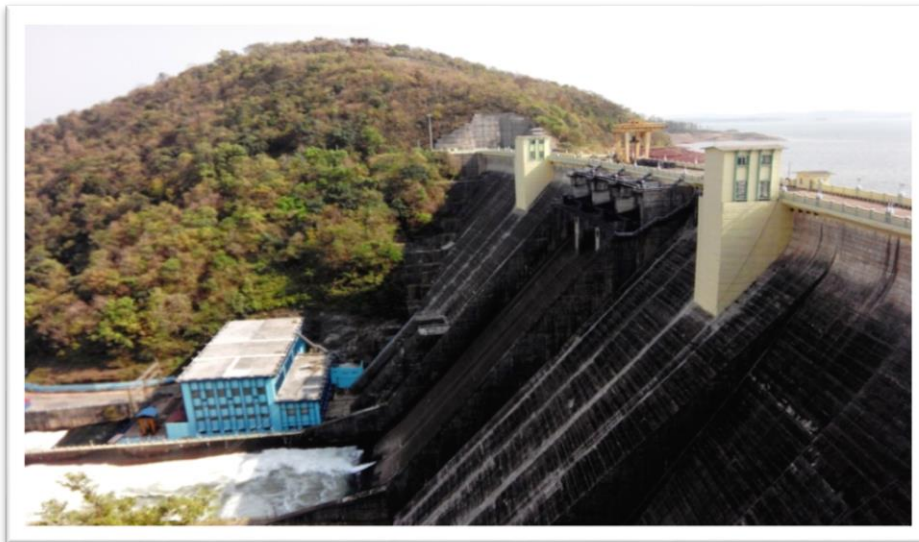
Supa dam and Power Station, Uttar Kannada
