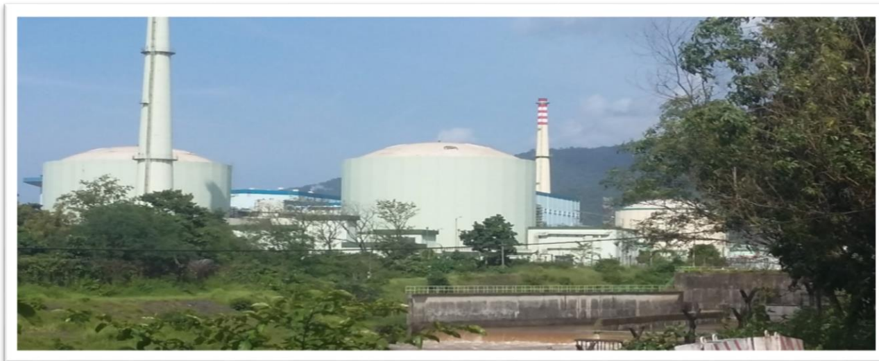
Kaiga Atomic Power Station, Uttar Kannada, Karnataka
